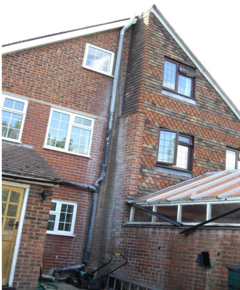
Figure 9. External view from neighbours side (NW) of rear addition/conservatory prior to rebuild works showing the high level windows recessed from the cavity wall.
